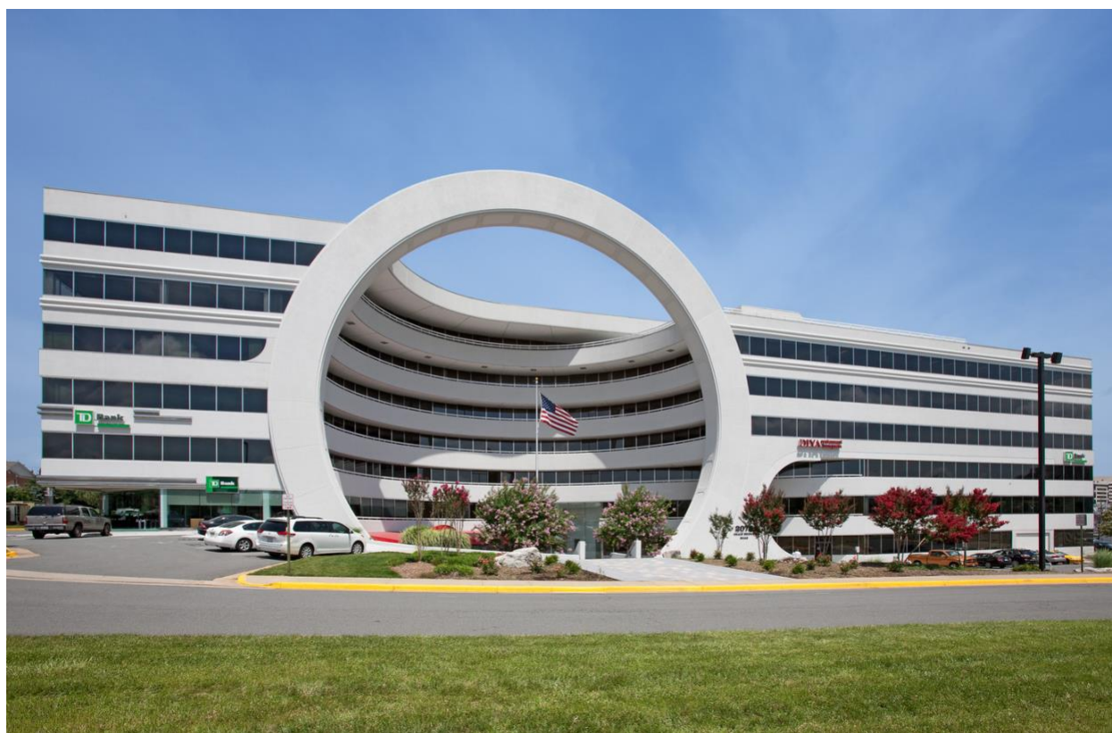
VUST Campus Building-Suite G100 (on the ground level)
